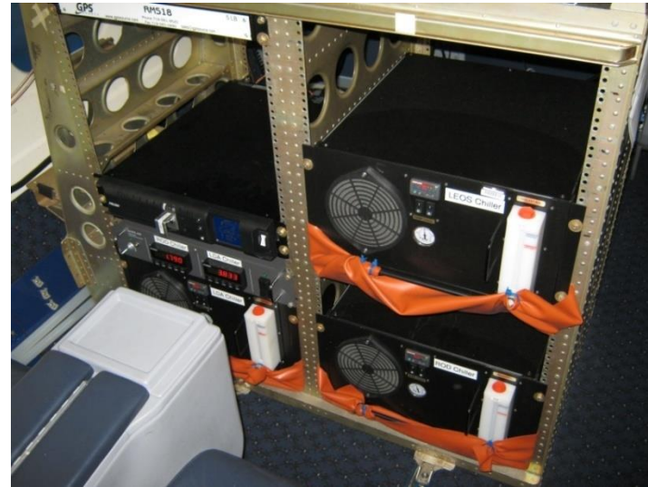
Laser Chillers in Passenger Level
