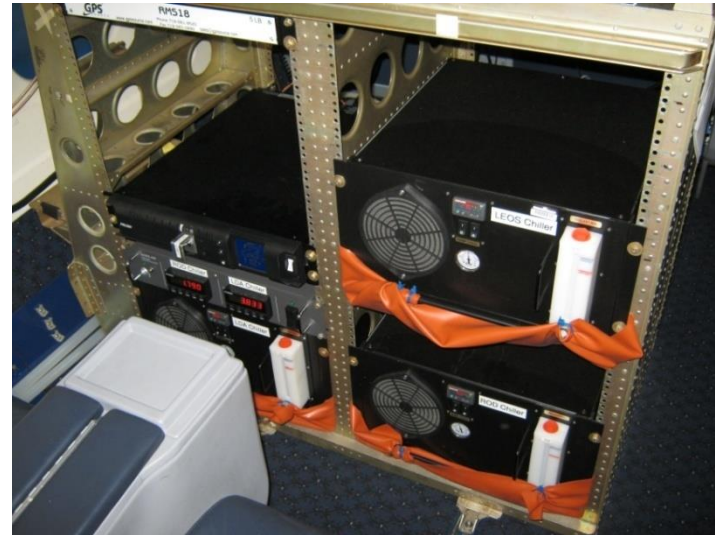
Laser Chillers in Passenger Level
